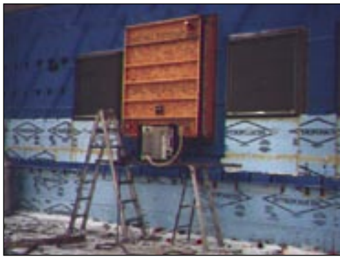
Figure 8: Testing a window enclosure and its perimeter joint using ASTM E 283.
