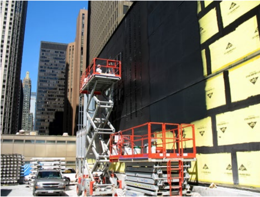
Photo courtesy Glen Trench/W.R. Meadows
