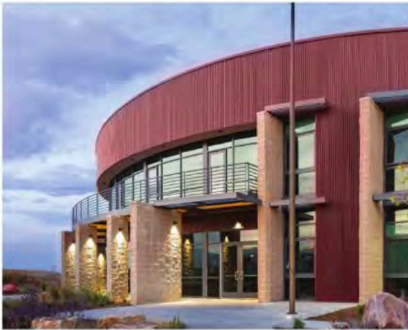
During the construction of the Boulder Wildland Fire Station in Boulder, Colorado, an air- and water-resistive barrier (AWB) system was selected for its high standard of durability.
