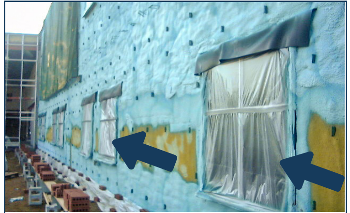
Typical masking off of windows prior to the installation of spray polyurethane foam.
