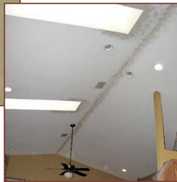
Figure 2. Water damage.
