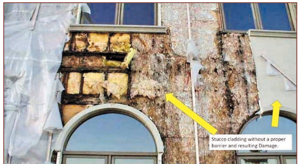
Figure 6. Wall damage.
