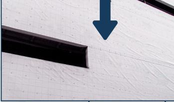
The overlapping of the sheet system and the location of the attachment discs need to be coordinated – air will get under the tape at the discs in these cases because of a lack of tape seal at and adjacent to the disc.
