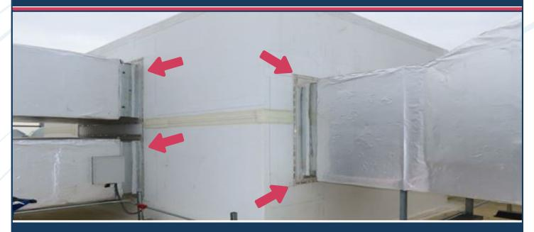
Several items to pay attention to is the ductwork is moving, expanding with temperature changes within the duct, air movement, etc. Those movements must be accommodated in the air barrier connection to the ductwork and penthouse. Also, review chemical and adhesion compatibility of materials to make the assembly.
