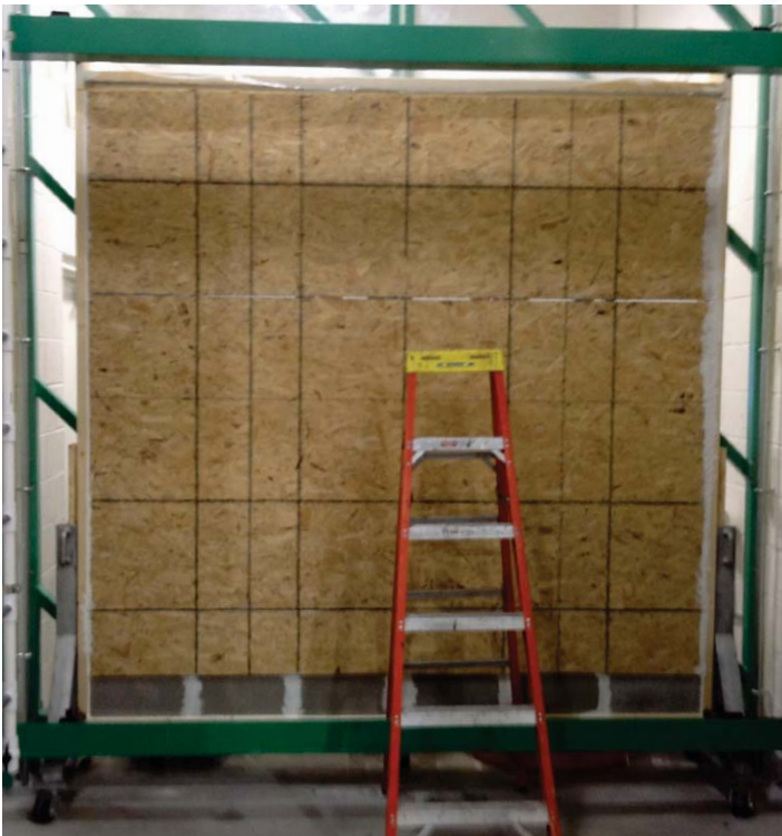
Figure 3: Test Wall Ready for Material Application
