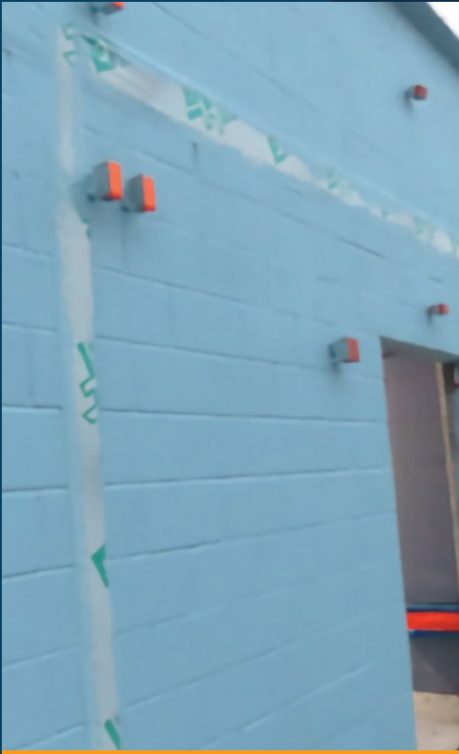
Installing liquid & peel and stick on CMU walls.
