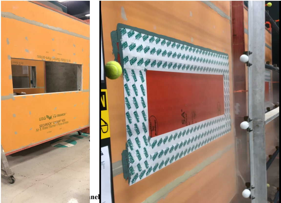
Figure 8: Wood buck with panel aperture (left) and panel installed (right).
